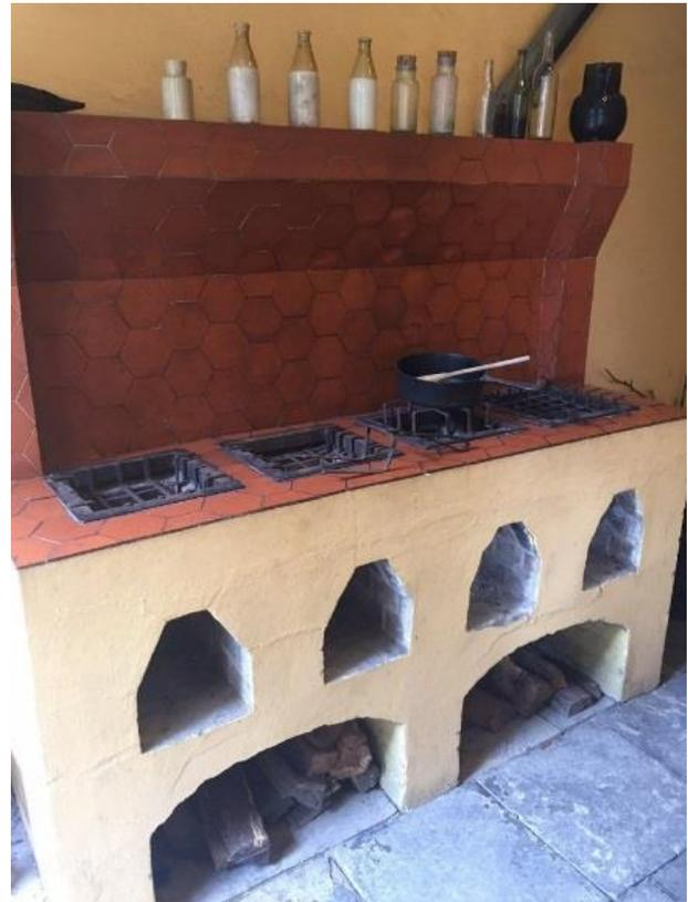
**The Four-Burner, Wood-Fire Stove with a Beehive Oven**
